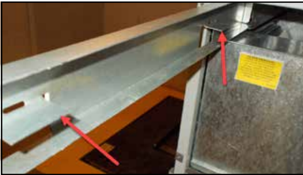
FIGURE 6 Remove Four Screws
