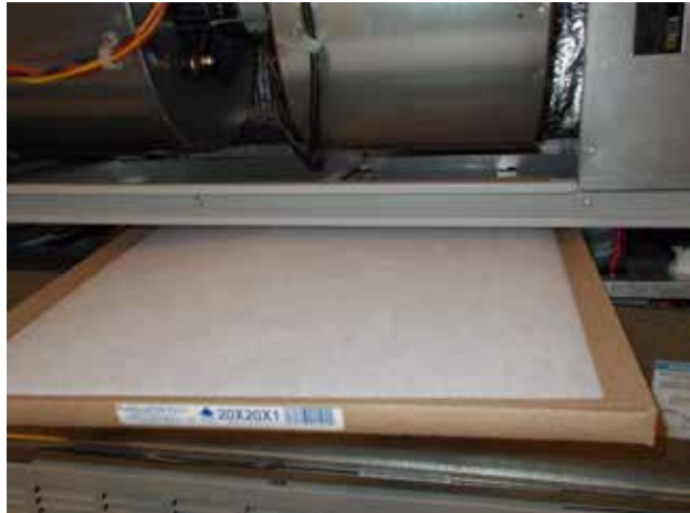
FIGURE 9 Install Left 1" Filter
