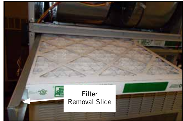
FIGURE 3 Removing Second Filter
