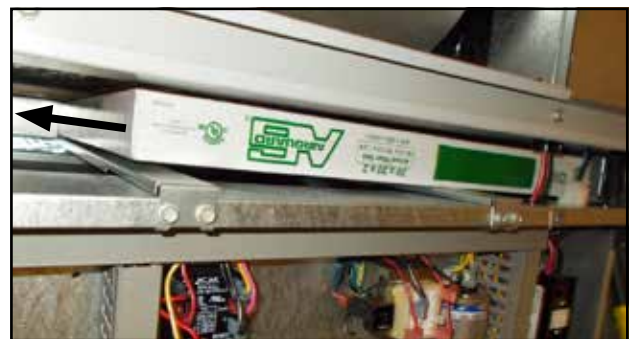
FIGURE 3 Removing Second Filter
