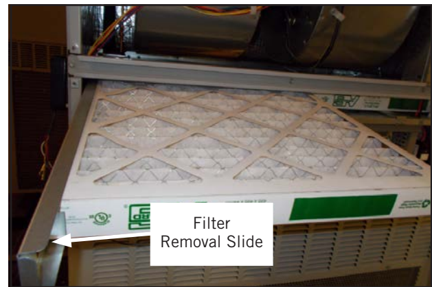
FIGURE 3 Removing Second Filter
