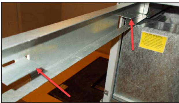
FIGURE 5 Bend Filter Tabs to Up Position
