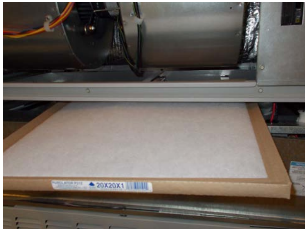
FIGURE 8 Install Right 1" Filter
