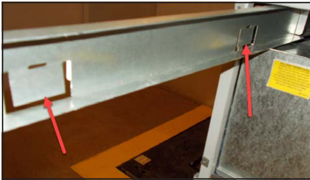
FIGURE 5 Bend Filter Tabs to Up Position
