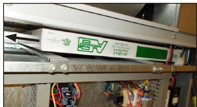
FIGURE 3 Removing Second Filter
