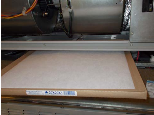
FIGURE 9 Install Left 1" Filter
