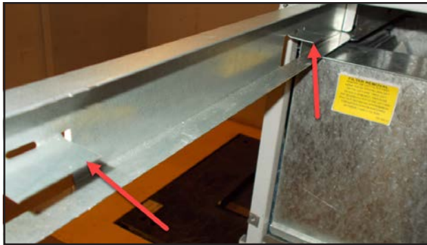
FIGURE 6 Remove Four Screws
