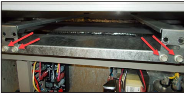
FIGURE 6 Remove Four Screws
