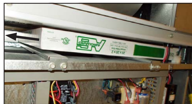
FIGURE 3 Removing Second Filter
