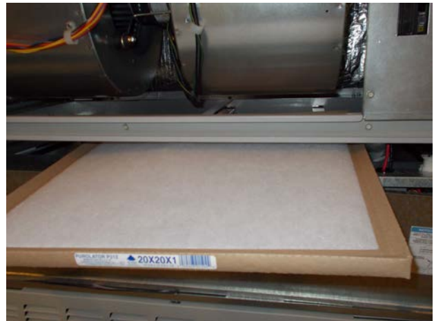
FIGURE 8 Install Right 1" Filter
