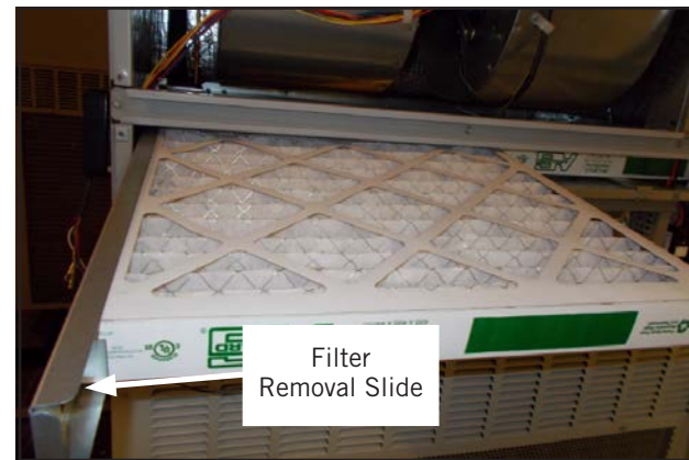
FIGURE 3 Removing Second Filter
