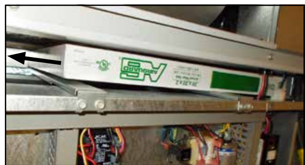
FIGURE 3 Removing Second Filter
