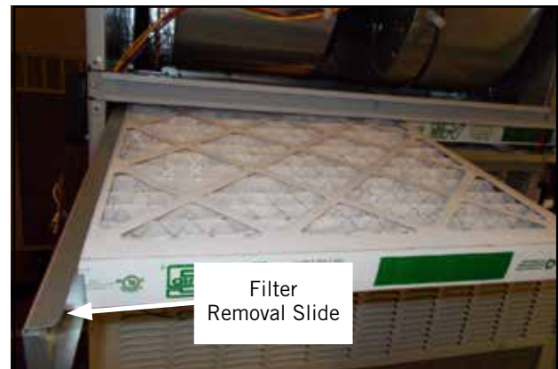
FIGURE 3 Removing Second Filter
