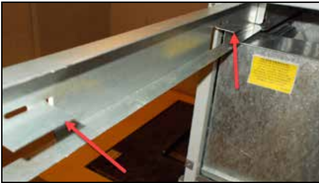
FIGURE 5 Bend Filter Tabs to Up Position
