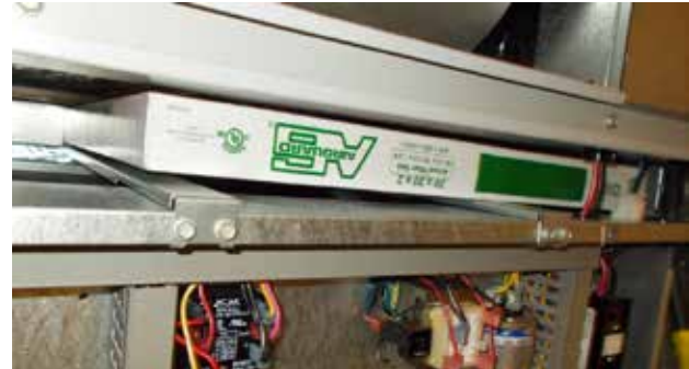
FIGURE 42 Install Left 2" Filter
