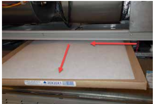
FIGURE 35 Removing Second Filter
