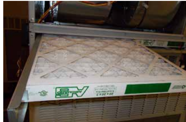
FIGURE 42 Install Left 2" Filter
