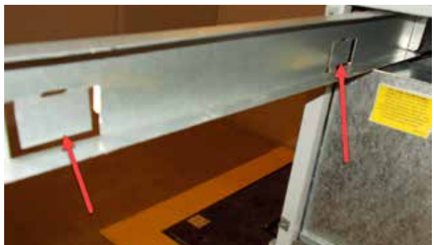
FIGURE 37 Bend Filter Tabs Down
