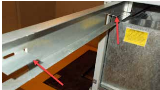
FIGURE 36 Filter Tabs in Up Position
