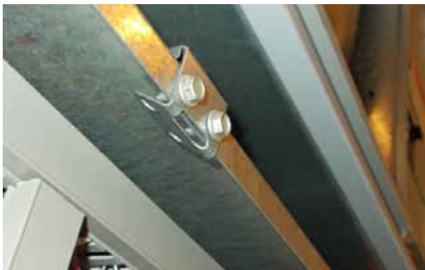
FIGURE 40 Re-Install Screws and Bend Tabs Up
