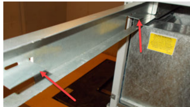
FIGURE 36 Filter Tabs in Up Position
