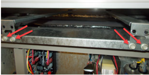
FIGURE 38 Remove Four Screws
