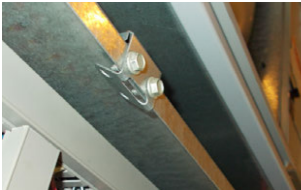
FIGURE 40 Re-Install Screws and Bend Tabs Up
