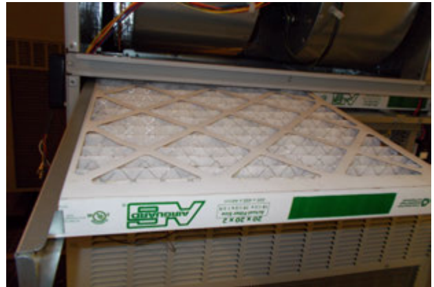
FIGURE 42 Install Left 2" Filter
