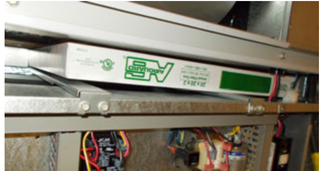
FIGURE 42 Install Left 2" Filter
