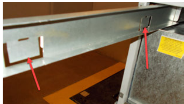
FIGURE 37 Bend Filter Tabs Down
