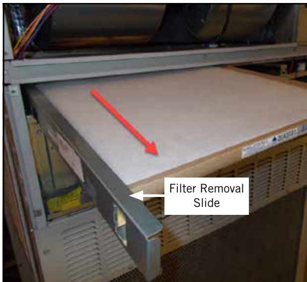
FIGURE 32 Removing Left Filter
