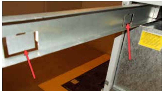
FIGURE 35 Bend Filter Tabs Down
