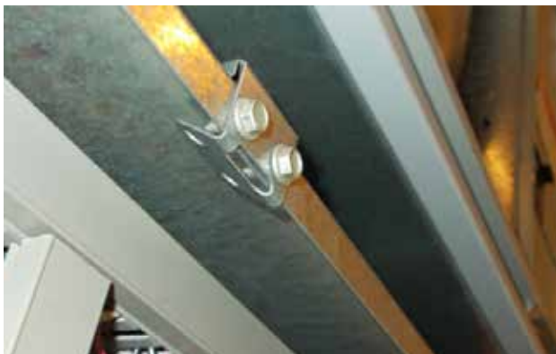
FIGURE 38 Re-Install Screws and Bend Tabs Up
