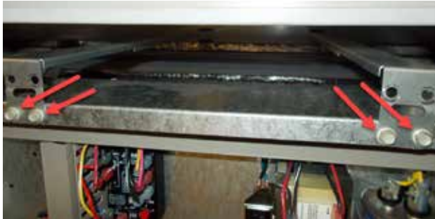
FIGURE 36 Remove Four Screws
