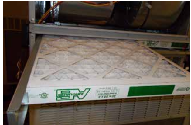
FIGURE 40 Install Left 2" Filter
