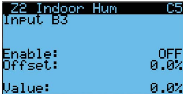
FIGURE 34 Enable/Disable Zone 2 Indoor Humidity Sensor
