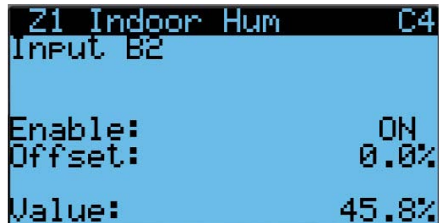
FIGURE 32 Enable/Disable Zone 1 Indoor Humidity Sensor
