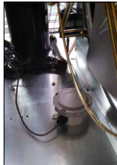
FIGURE 3 Outdoor Sensor Installation
