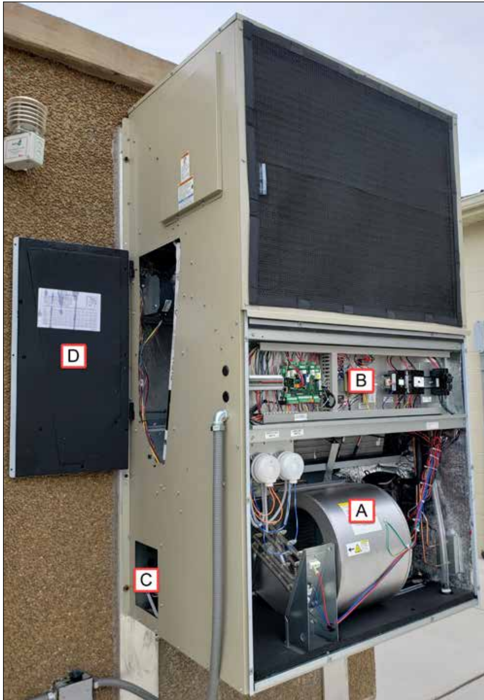
FIGURE 1 Wall Unit Panels
