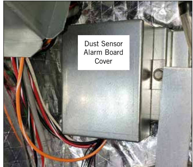
FIGURE 4 Remove Dust Sensor Alarm Board Cover
