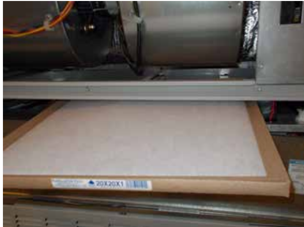
FIGURE 9 Install Left 1" Filter
