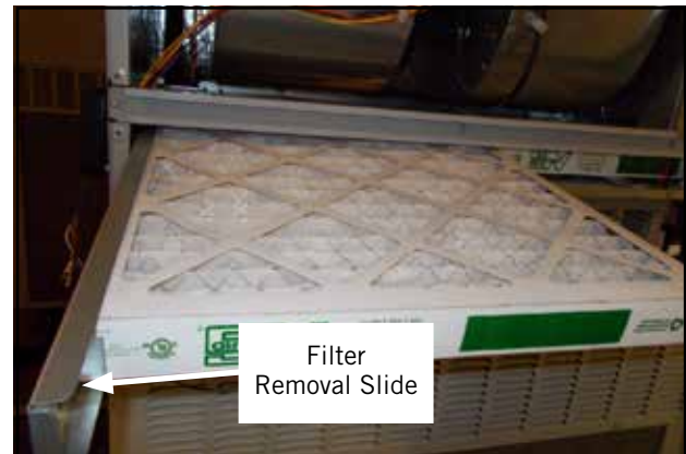
FIGURE 3 Removing Second Filter
