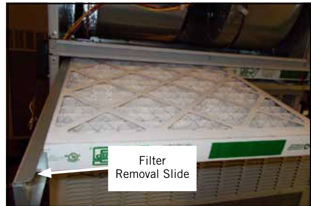
FIGURE 3 Removing Second Filter
