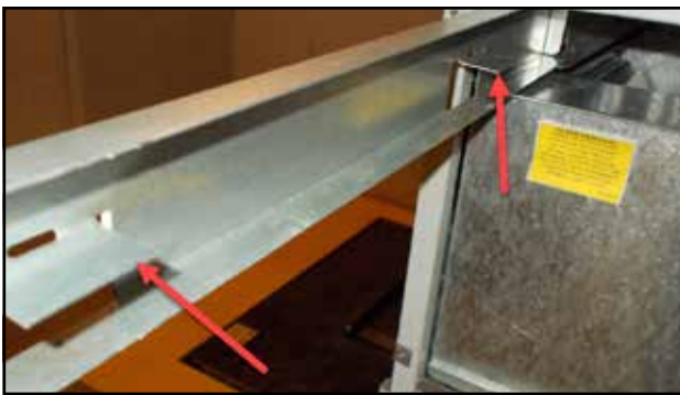
FIGURE 5 Bend Filter Tabs to Up Position
