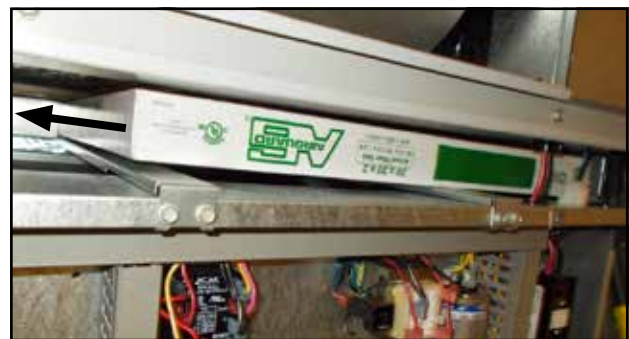
FIGURE 3 Removing Second Filter
