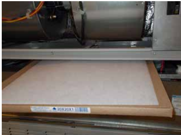
FIGURE 8 Install Right 1" Filter
