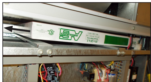
FIGURE 3 Removing Second Filter
