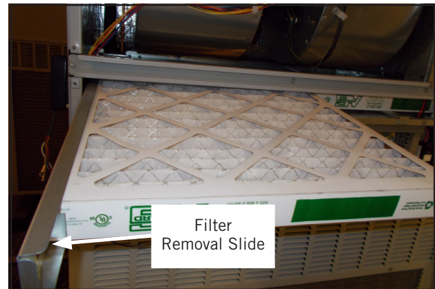
FIGURE 3 Removing Second Filter
