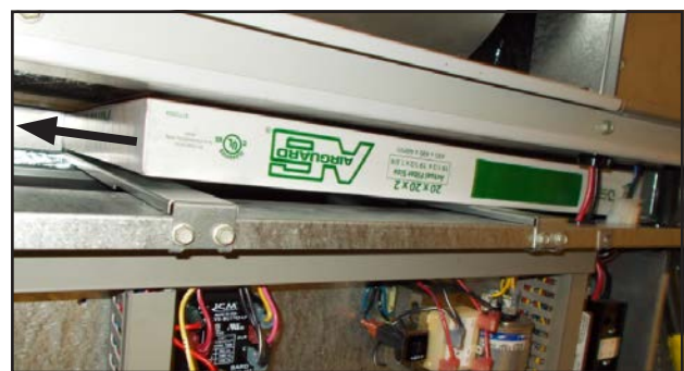
FIGURE 3 Removing Second Filter
