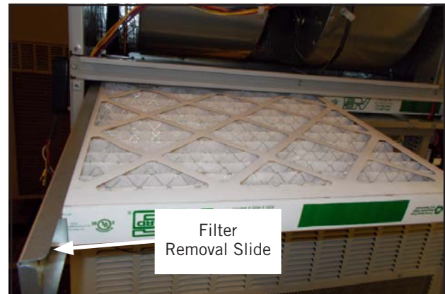
FIGURE 3 Removing Second Filter
