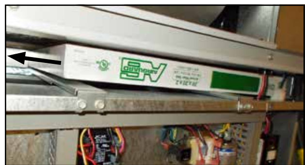
FIGURE 3 Removing Second Filter
