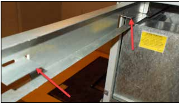
FIGURE 5 Bend Filter Tabs to Up Position
