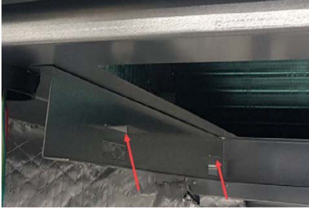
FIGURE 10 Bend Filter Tabs Down
