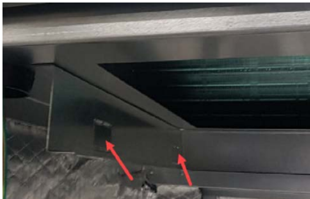
FIGURE 10 Bend Filter Tabs Down
