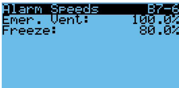
FIGURE 29 Adjusting Emergency Vent and Freeze Speeds
