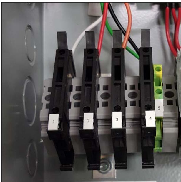
FIGURE 15 LC6000 Fused Power Supply Terminal
