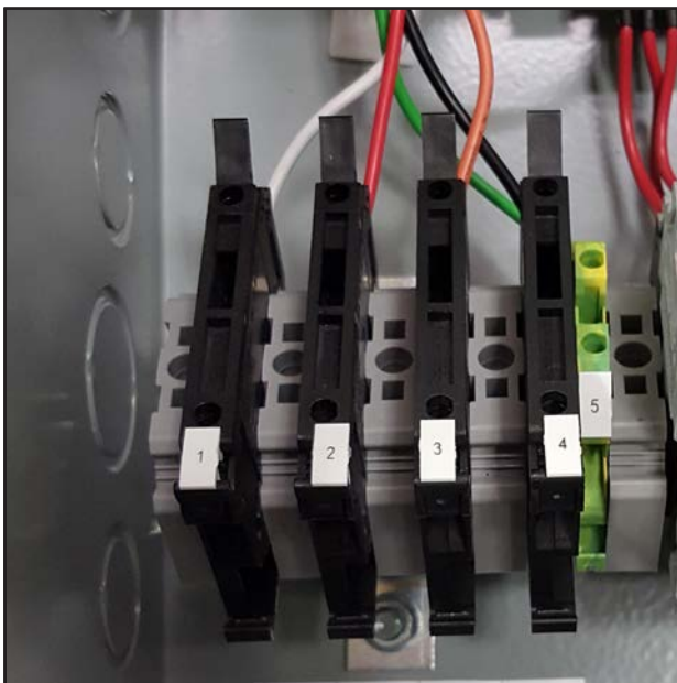
FIGURE 15 LC6000 Fused Power Supply Terminal
