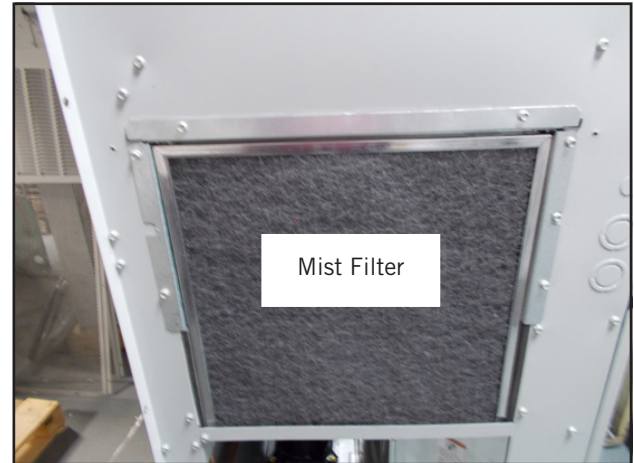
FIGURE 16 Install Mist Filters
