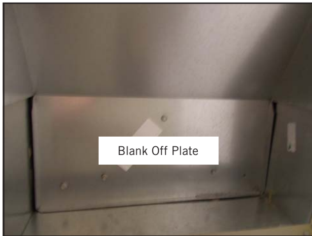
FIGURE 4 Remove Blank Off Plates (Both Sides)
