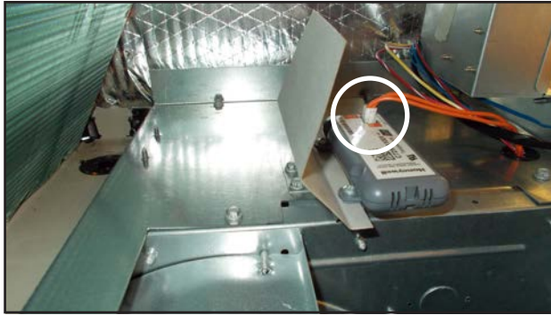
FIGURE 16 Connect Mixed Air Sensor Plug
