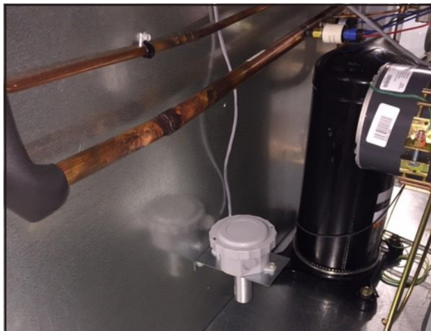
FIGURE 18 Temperature Only Sensor Assembly Installation
