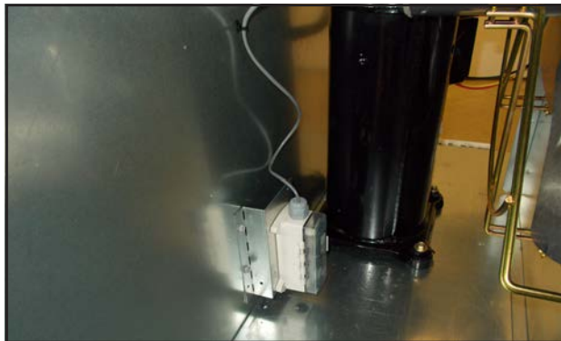
FIGURE 17 Enthalpy Sensor Assembly Installation
