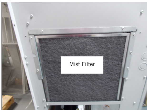
FIGURE 26 Install Mist Filters
