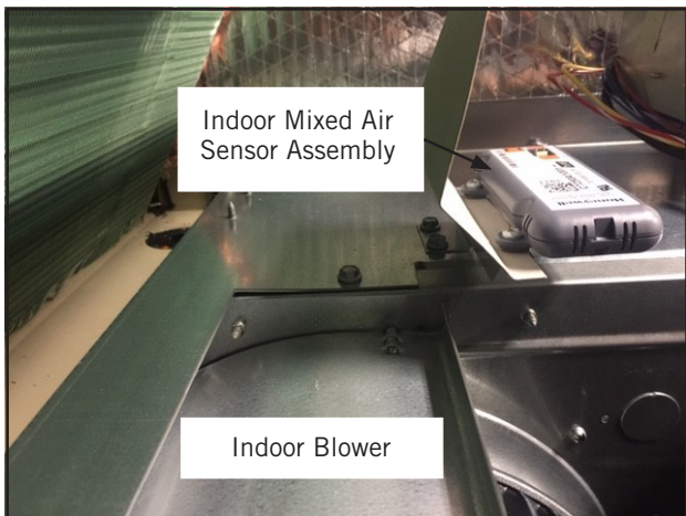
FIGURE 13 Install Indoor Mixed Air Sensor Assembly
