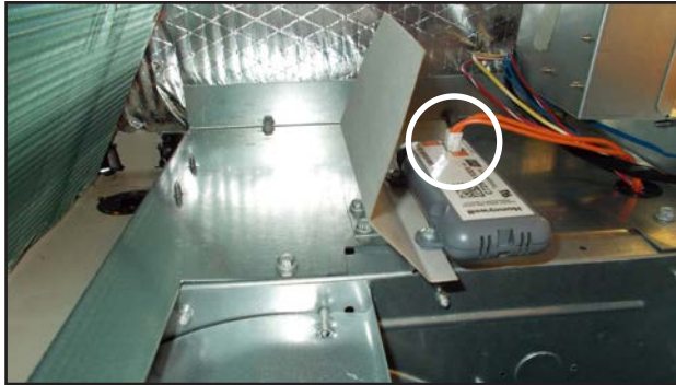
FIGURE 16 Connect Mixed Air Sensor Plug
