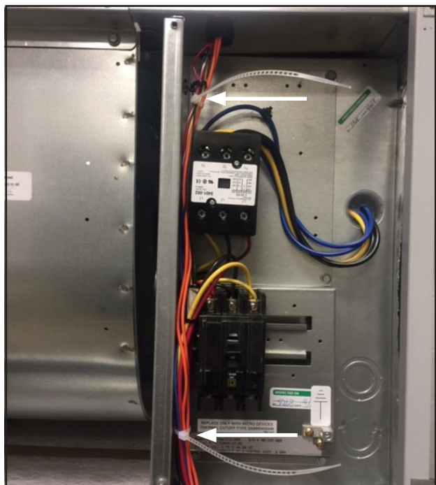
FIGURE 15 Secure Sensor Wires with Ladder Ties
