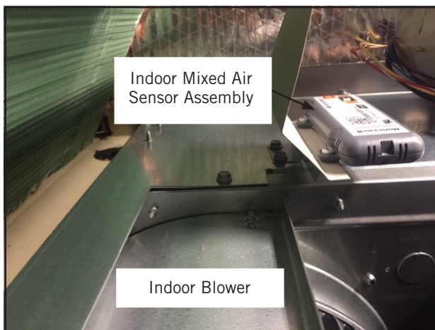
FIGURE 13 Install Indoor Mixed Air Sensor Assembly
