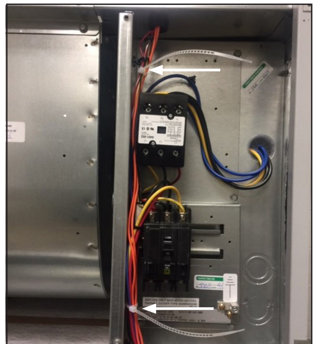
FIGURE 15 Secure Sensor Wires with Ladder Ties
