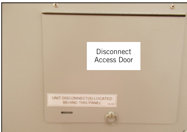
FIGURE 1 Disconnect Power
