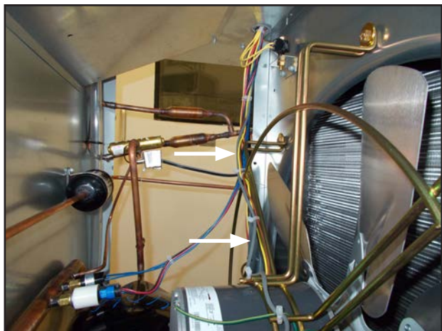
FIGURE 19 Route Wires and Secure with Ties
