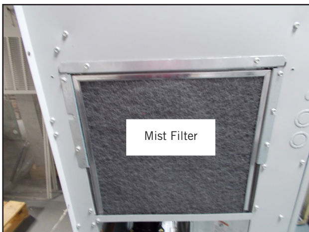
FIGURE 26 Install Mist Filters
