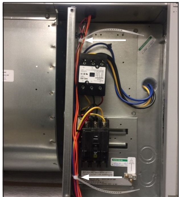
FIGURE 15 Secure Sensor Wires with Ladder Ties
