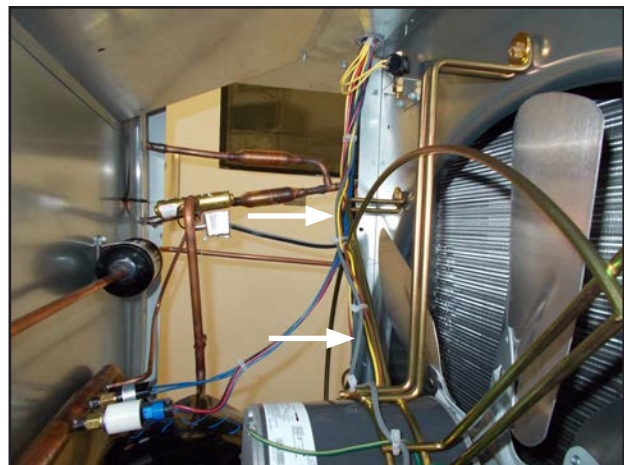
FIGURE 19 Route Wires and Secure with Ties
