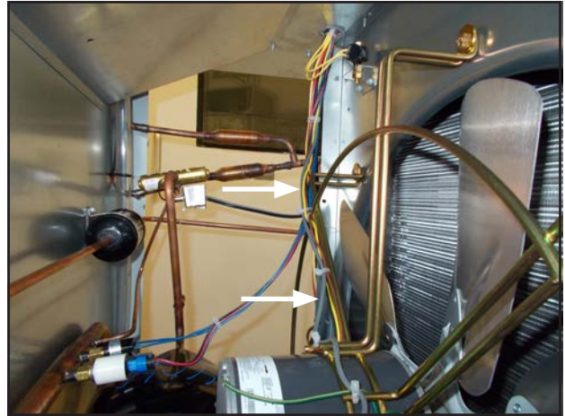
FIGURE 19 Route Wires and Secure with Ties
