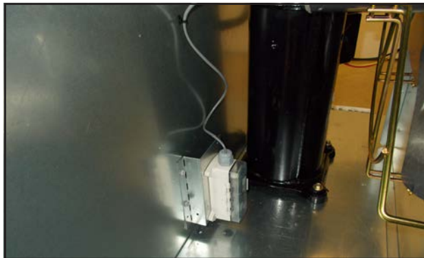
FIGURE 17 Enthalpy Sensor Assembly Installation
