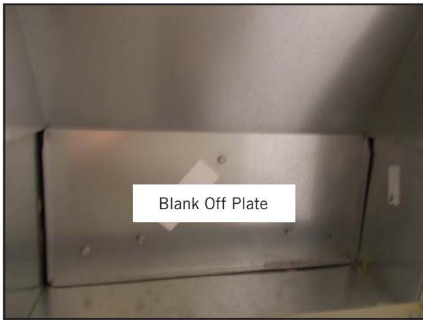
FIGURE 4 Remove Blank Off Plates (Both Sides)
