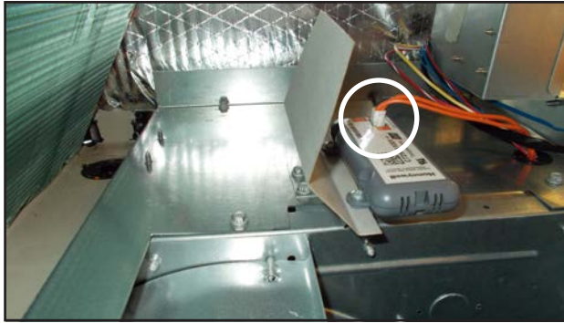
FIGURE 16 Connect Mixed Air Sensor Plug
