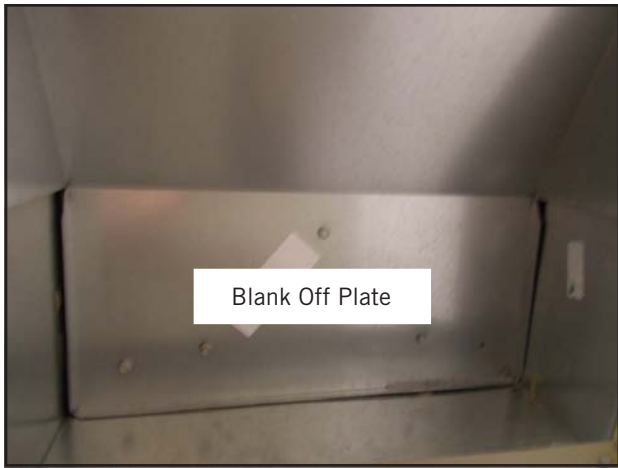
FIGURE 4 Remove Blank Off Plates (Both Sides)
