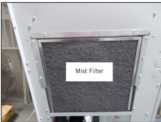
FIGURE 14 Install Mist Filters
