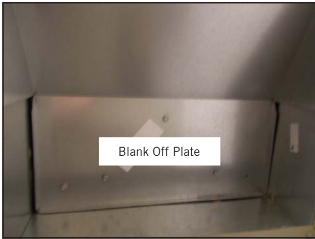
FIGURE 4 Remove Blank Off Plates (Both Sides)
