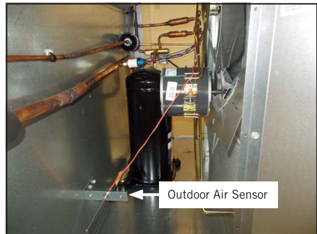
FIGURE 7 Install Outdoor Air Sensor
