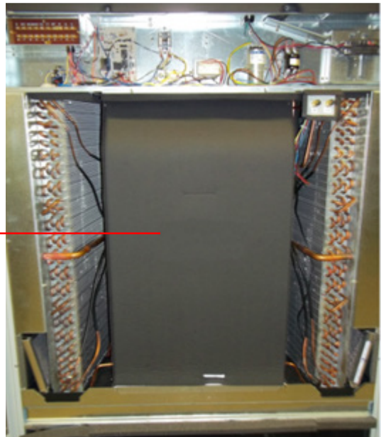
FIGURE 6 Removal of Air Duct
