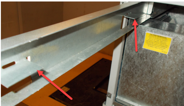
FIGURE 4 Filter Tabs in Up Position
