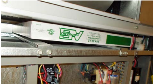
FIGURE 10 Install Left 2" Filter
