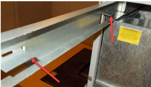
FIGURE 4 Filter Tabs in Up Position (1" Filter)
