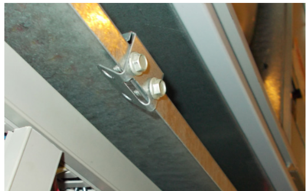
FIGURE 8 Re-Install Screws and Bend Tabs Up
