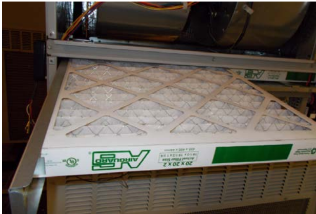
FIGURE 10 Install Left 2" Filter
