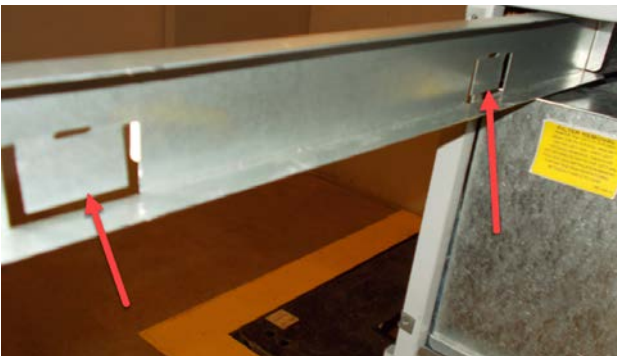
FIGURE 5 Bend Filter Tabs Down (2" Filter)
