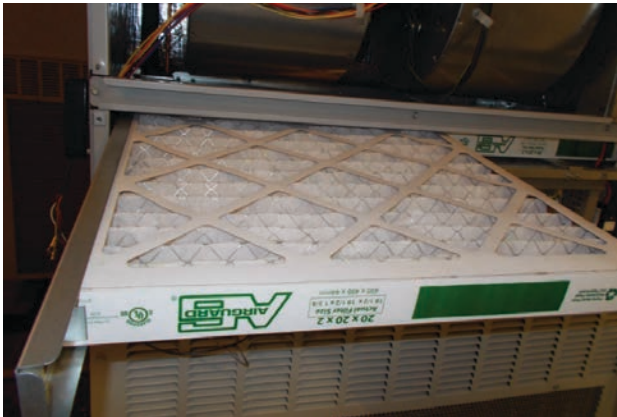
FIGURE 10 Install Left 2" Filter
