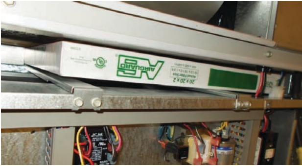
FIGURE 10 Install Left 2" Filter
