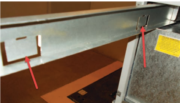
FIGURE 5 Bend Filter Tabs Down
