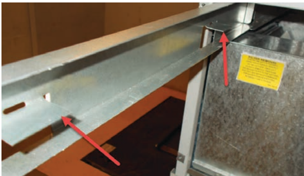
FIGURE 4 Filter Tabs in Up Position
