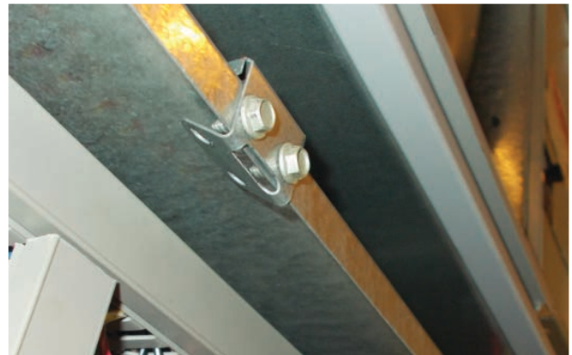
FIGURE 8 Re-Install Screws and Bend Tabs Up
