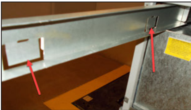
FIGURE 62 Bend Filter Tabs Down
