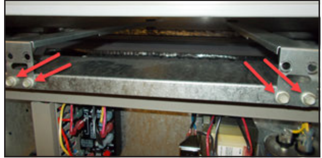
FIGURE 63 Remove Four Screws
