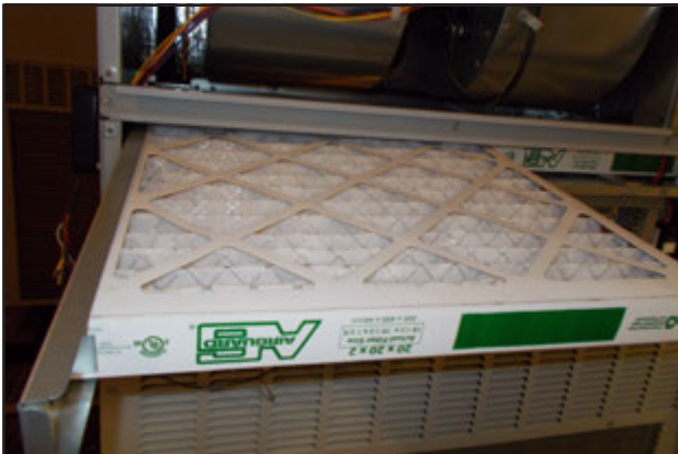
FIGURE 67 Install Left 2" Filter
