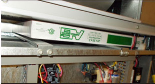
FIGURE 66 Install Right 2" Filter
