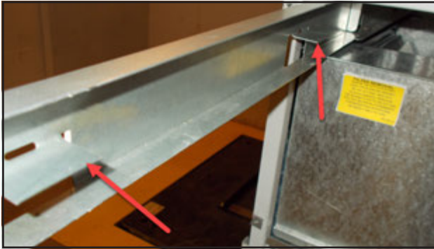
FIGURE 61 Filter Tabs in Up Position
