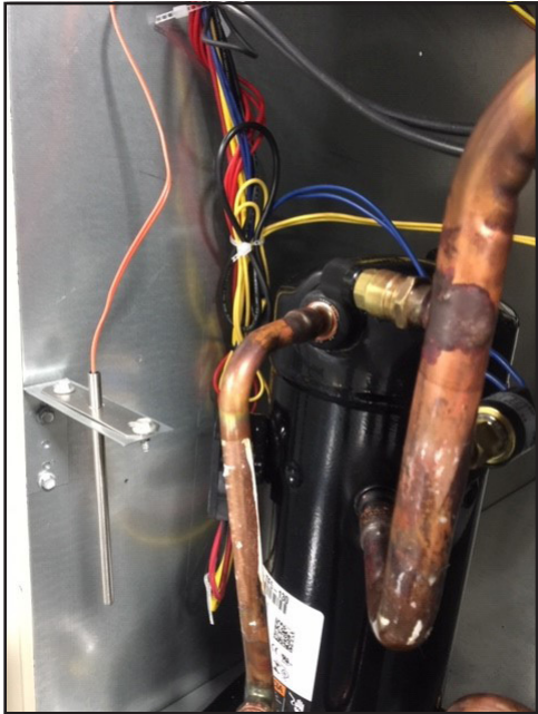
FIGURE 4 Outdoor Air Sensor Installation
