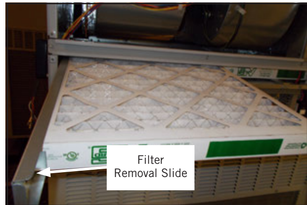
FIGURE 3 Removing Second Filter
