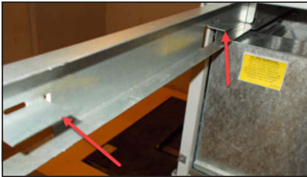
FIGURE 5 Bend Filter Tabs to Up Position
