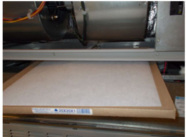
FIGURE 8 Install Right 1" Filter
