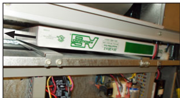
FIGURE 3 Removing Second Filter
