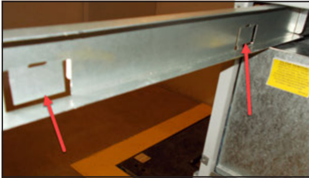
FIGURE 5 Bend Filter Tabs to Up Position
