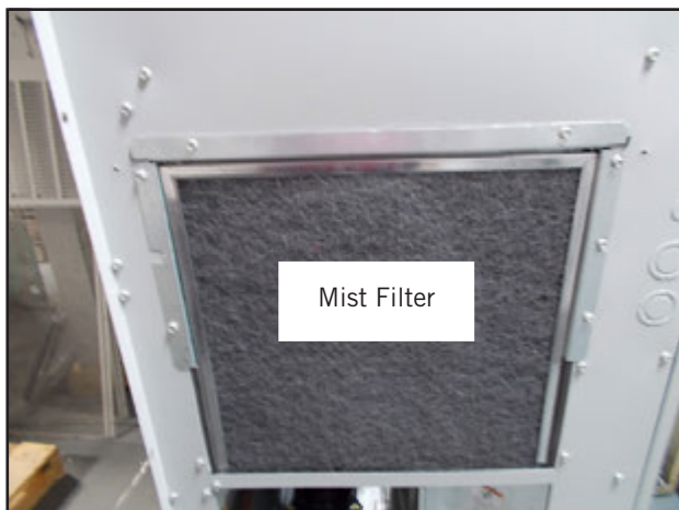
FIGURE 13 Install Mist Filters
