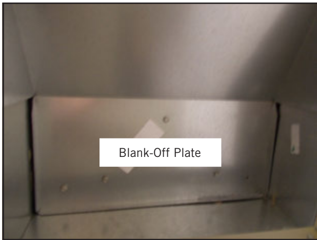
FIGURE 4 Remove Blank-Off Plates (Both Sides)
