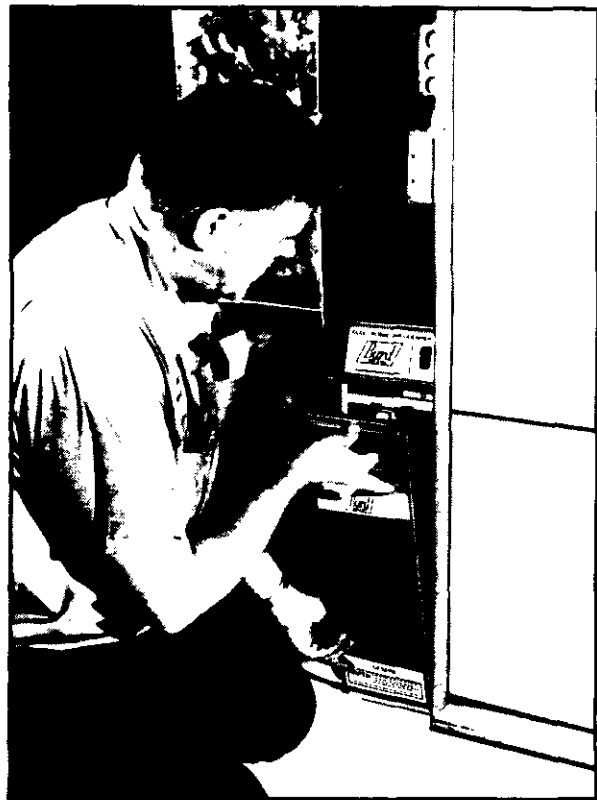
FIG. 28—CLOSE ACCESS DOOR TO COMPLETE AIR CLEANER INSTALLATION.
