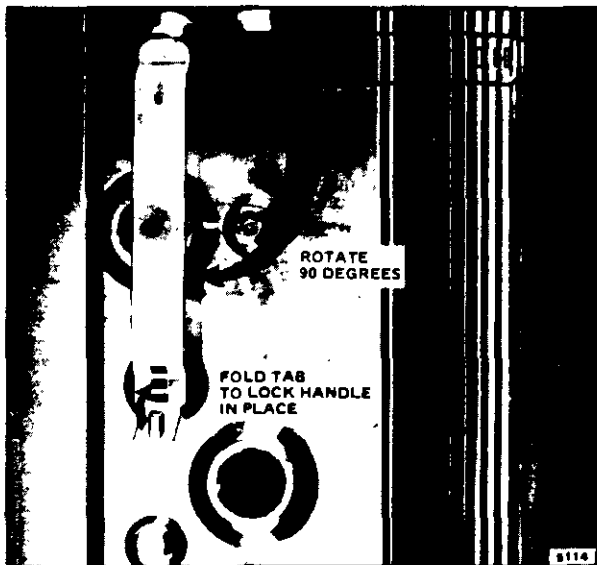
FIG. 27—INSTALL HANDLE ON END OF CELL THAT WILL BE CLOSEST TO ACCESS DOOR.
